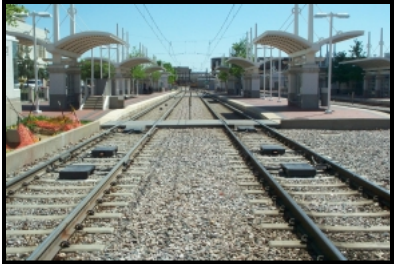
Signal Track Circuit Equipment at Union Station (OC-1 Area)
