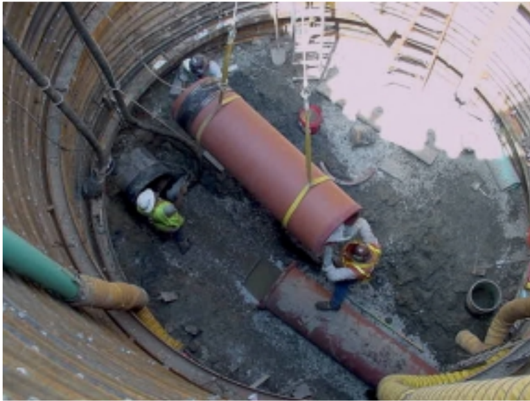
Replacement of Sanitary Sewer Pipe at OC-1 Junction Area
