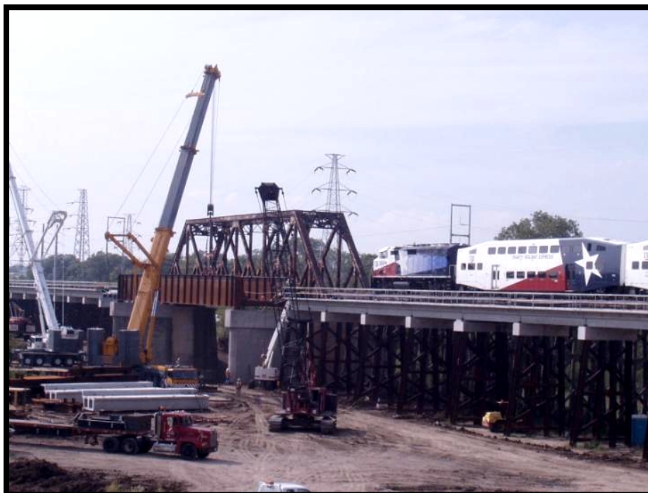
Girder Placement on South Bridge
