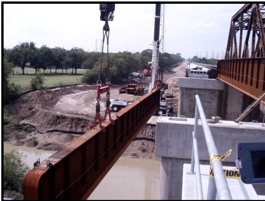
Girder Placement on South Bridge
