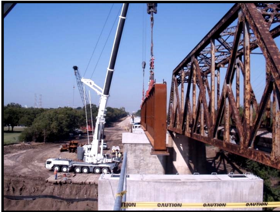
Girder Placement on South Bridge
