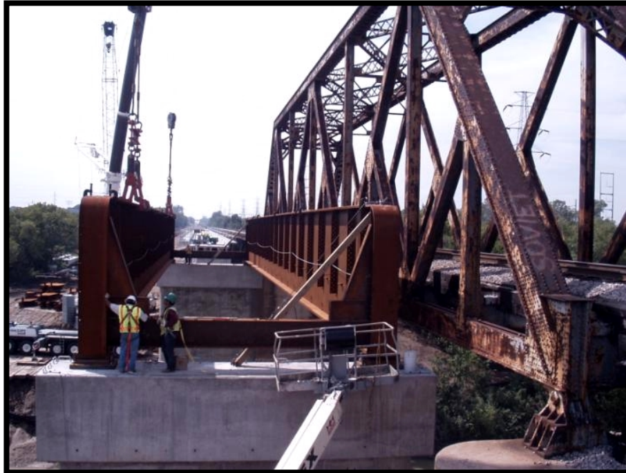
Girder Placement on South Bridge
