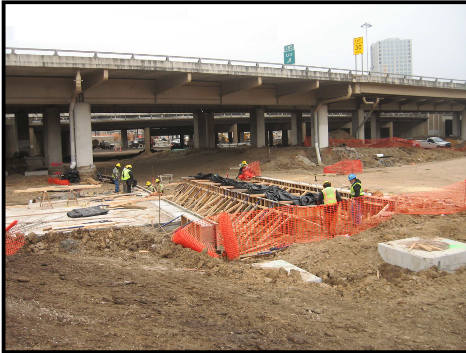
Forming Header at NB Central Service Road
