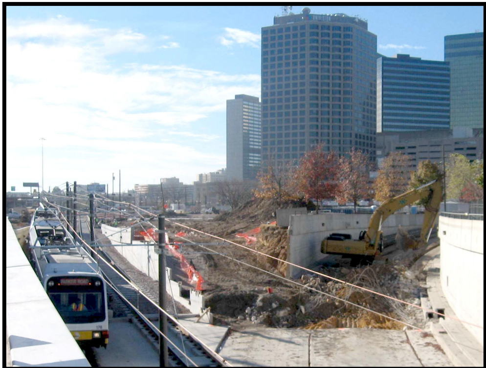
Demolition of Old Portal Track
