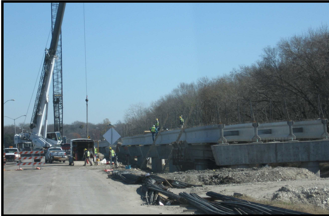
SE-2: Hanging Beams at White Rock Creek
