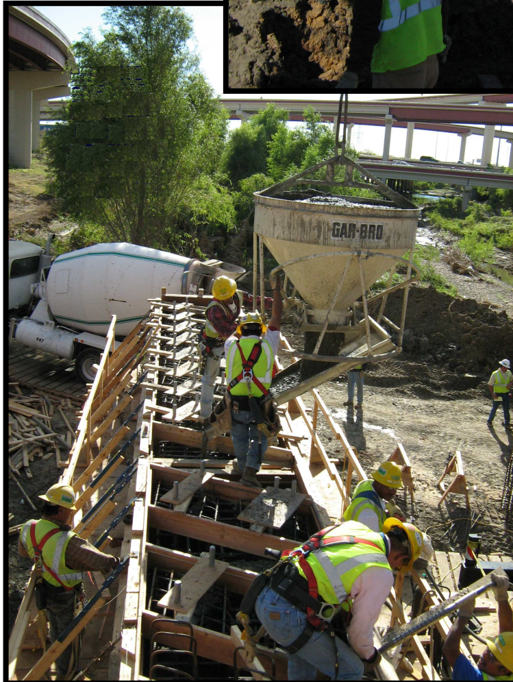
NW-4: Placing Concrete Pier Cap at Furneaux Creek
