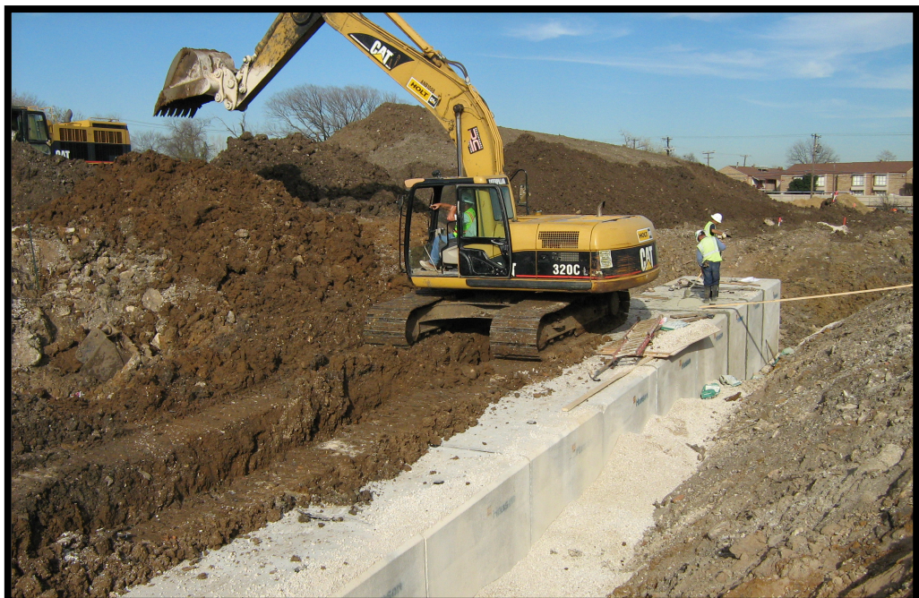
NW-2: Bachman Station Box Culvert
