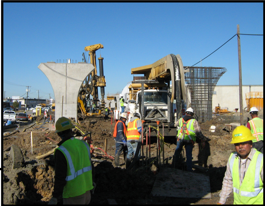
NW-3: Concrete Placement of Royal Lane Station Piers
