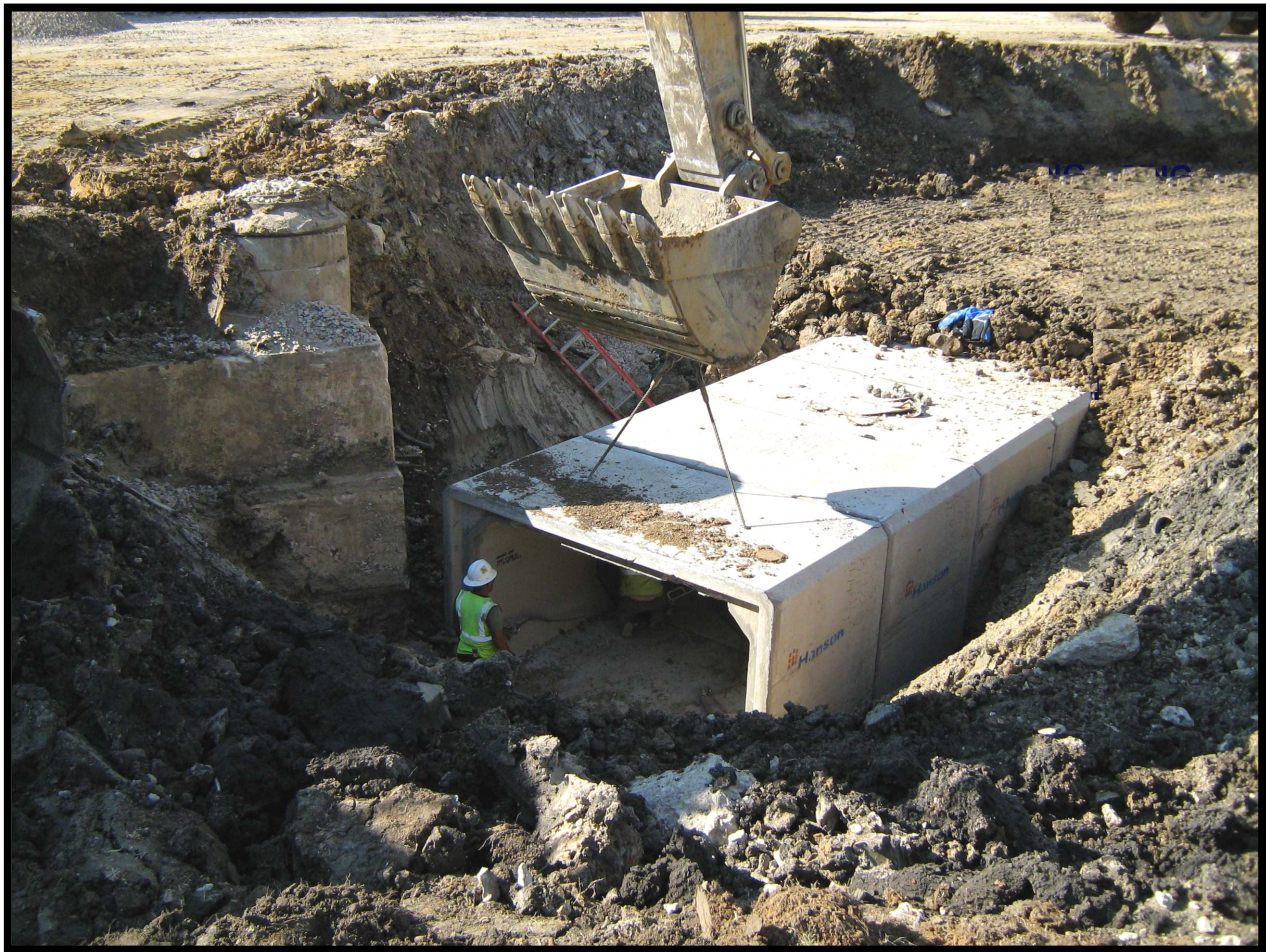
NW-4: Placing Box Culvert at Squire Place
