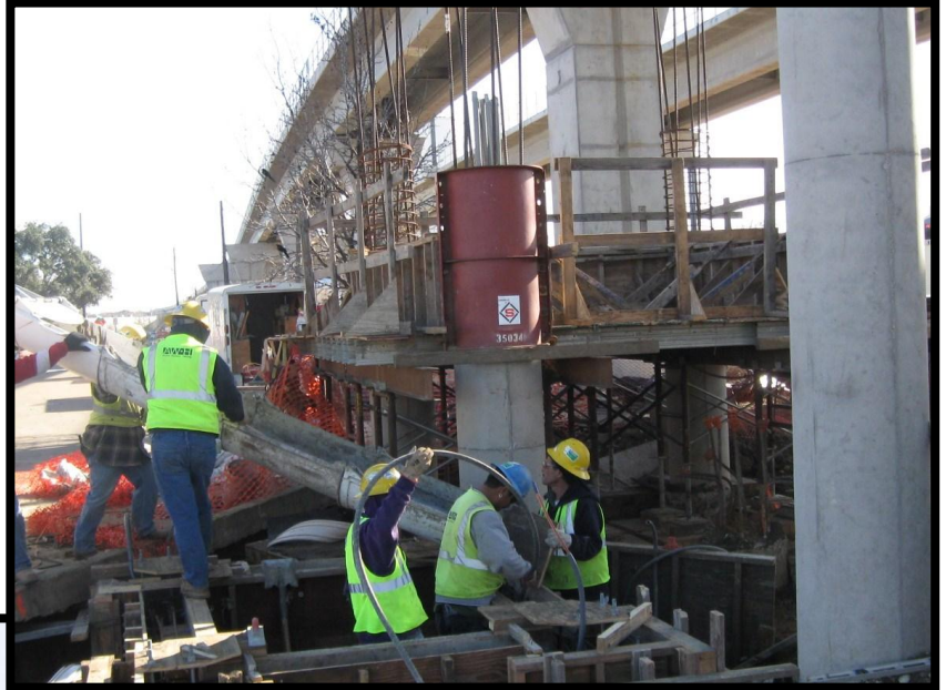
NW-4: Concrete Placement for Pedestrian Bridge Footing at Downtown Carrollton Station
