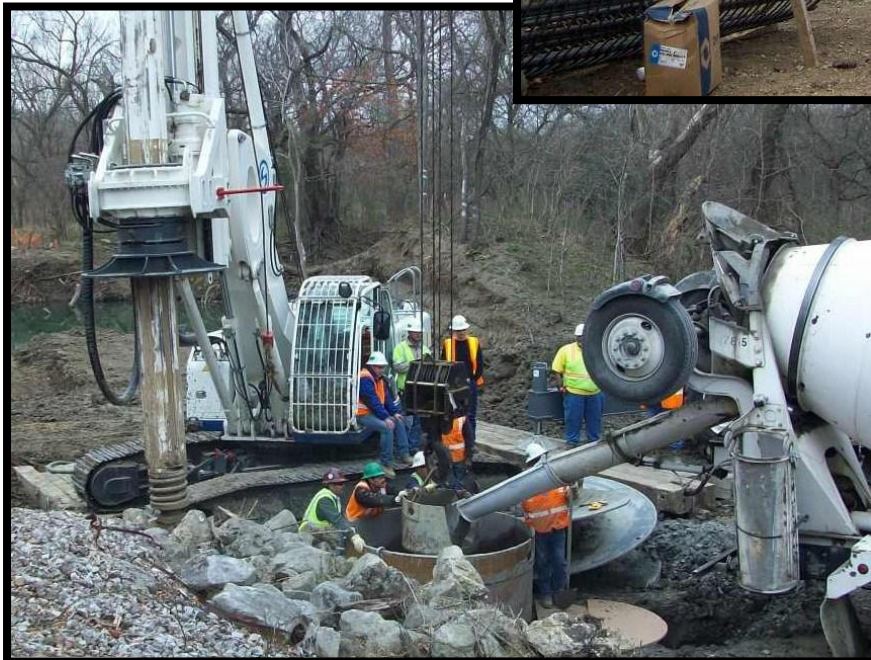
Concrete Placement for Drilled Shaft
