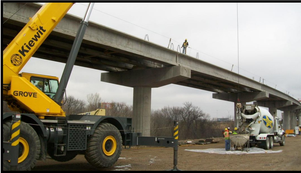
Placement of Shear Block
