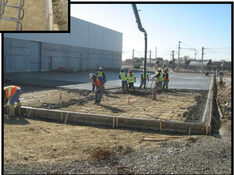
Placement of Concrete for WSA Parking Area
