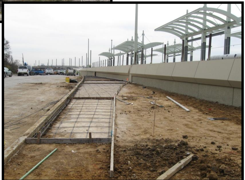
NW-2: Bachman Station Sidewalk Installation
