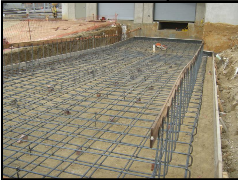
Rebar for WSA Loading Dock
