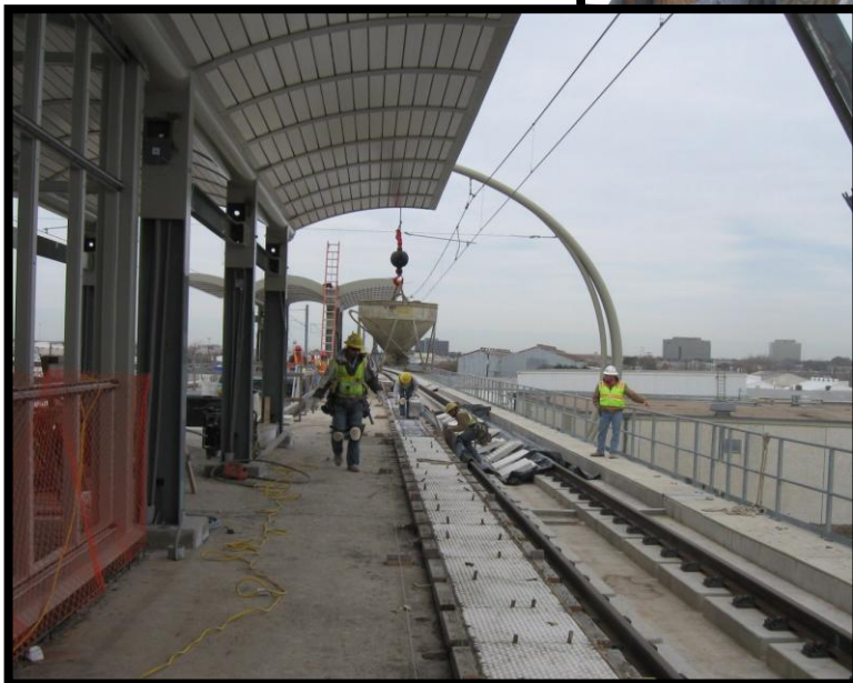
NW-3: Installation of Warning Strips at Royal Lane Station
