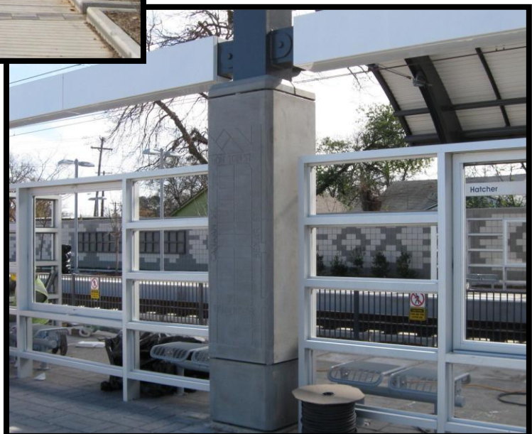
SE-1: Hatcher Station Column Cladding
