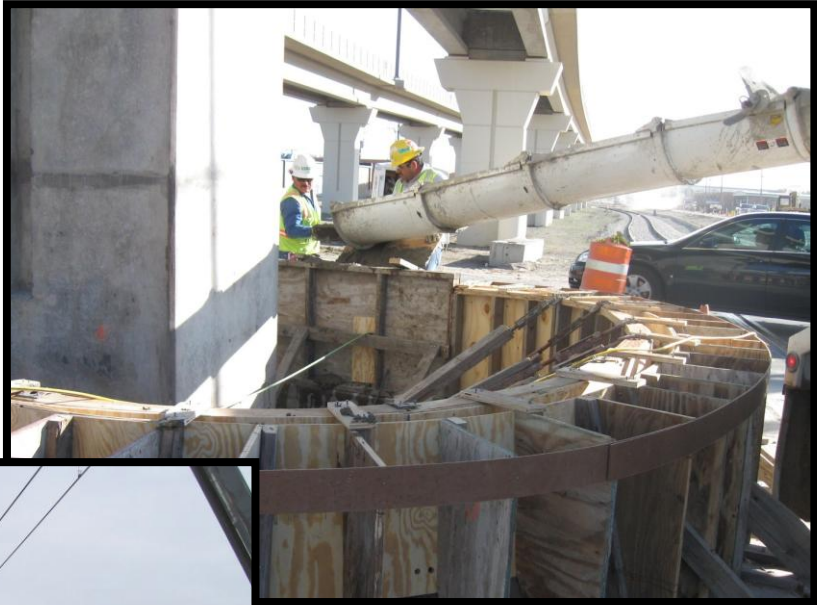
NW-3: Installation of Barrier Wall at Walnut Hill Lane
