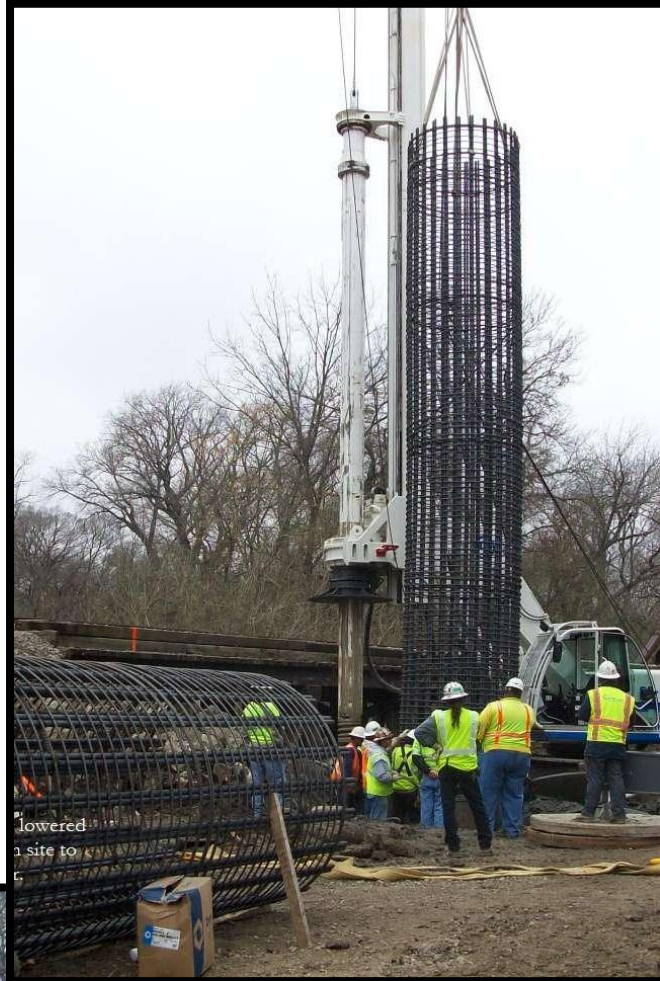
Rebar Cage Being Lowered into Hole
