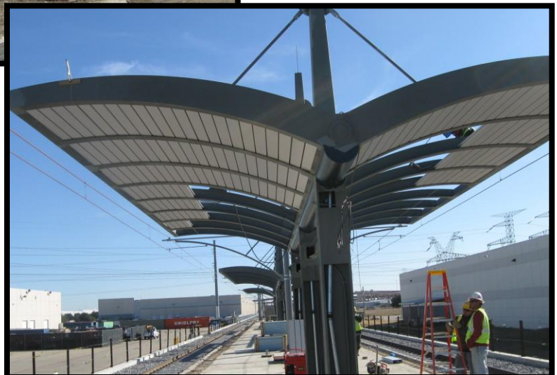
NW-3: Canopy Fascia Installation at North Carrollton/Frankford Station
