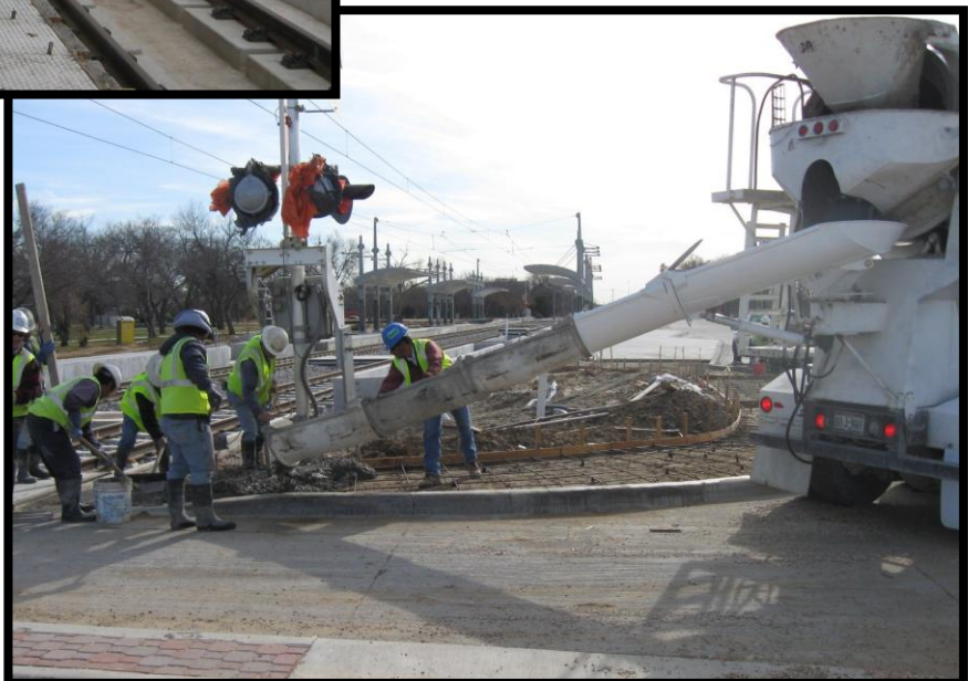
NW-3: Concrete Placement for Sidewalk near Farmers Branch Station
