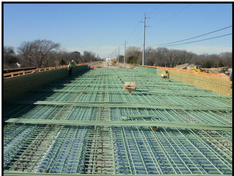
Deck Reinforcement at SH66 LRT Bridge
