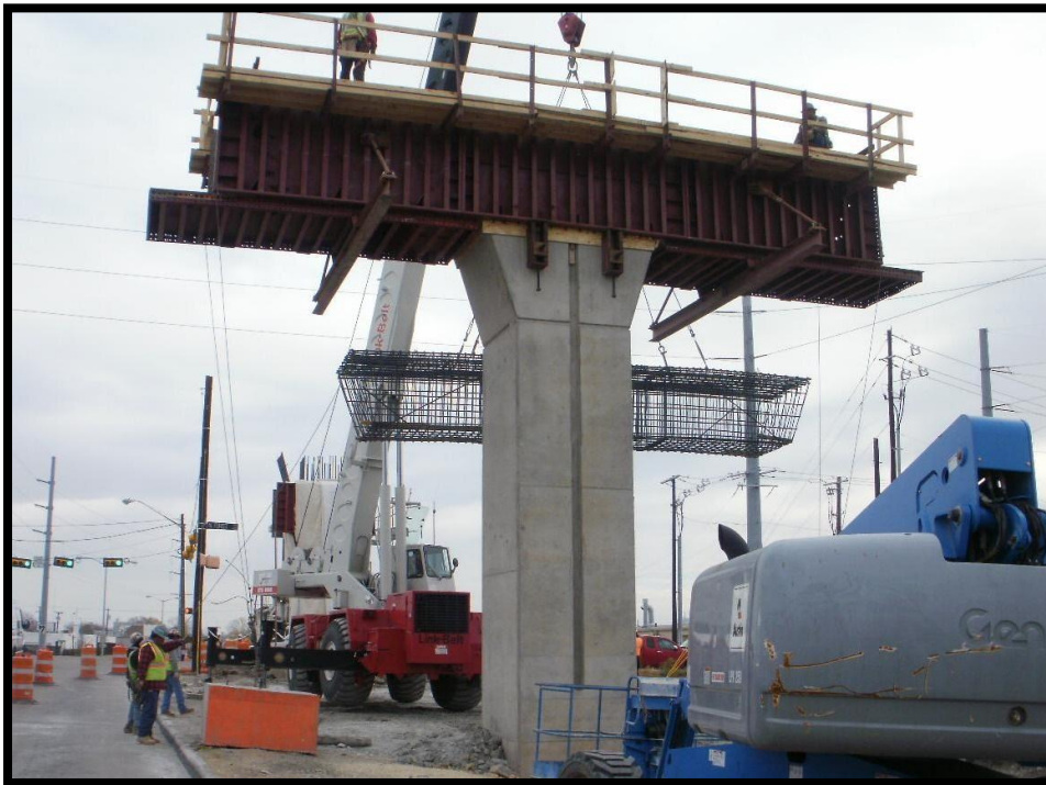
Bent Cap Construction at KCS Bridge
