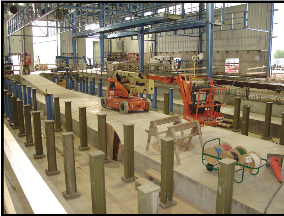
Pits, Pedestals, and Overhead Platforms in the Running Maintenance Extension
