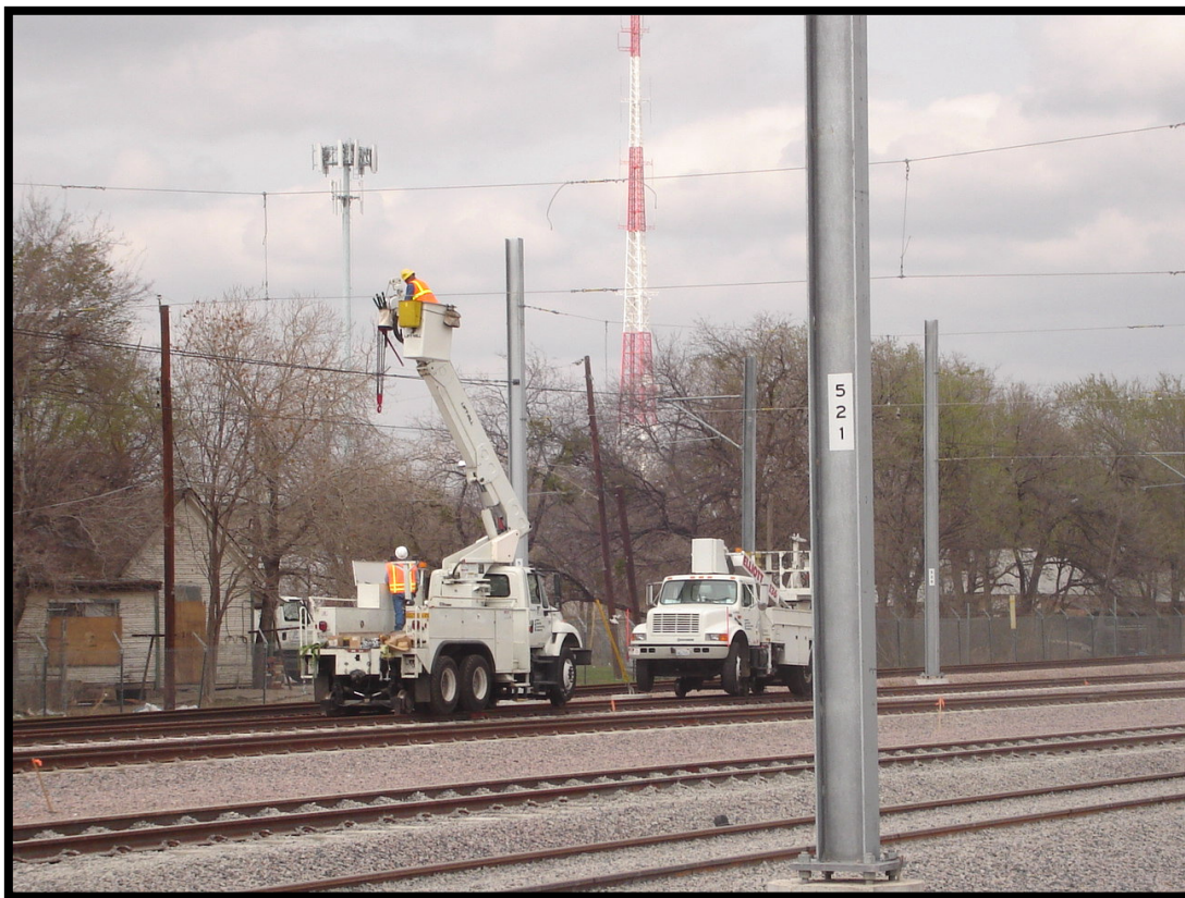
OCS Installation in Storage Track Area
