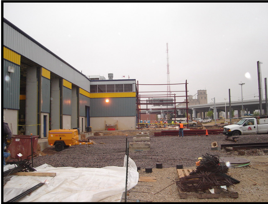
Bi-fold Doors of Running Maintenance Extension & Structural Steel at Body Shop
