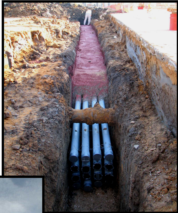
Duct Bank Installation
