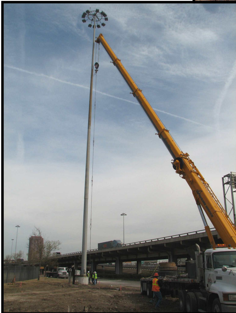
High Mast Lighting Relocation
