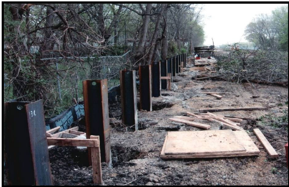
SE-2: H-Pile Wall Installation
