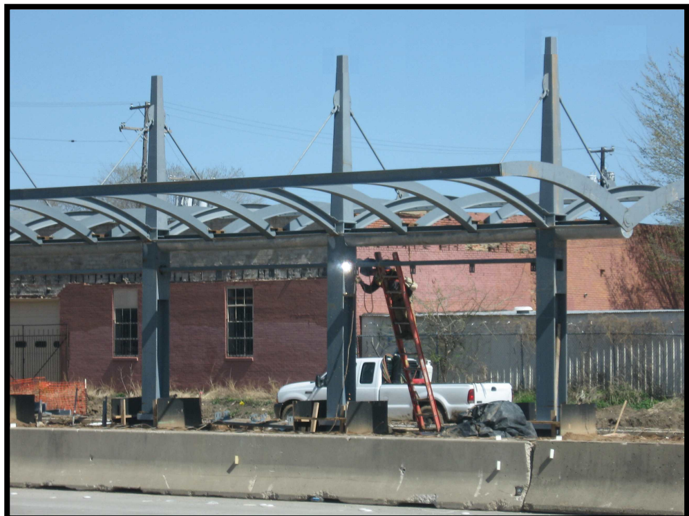
SE-1: Deep Ellum Station Canopy Welding
