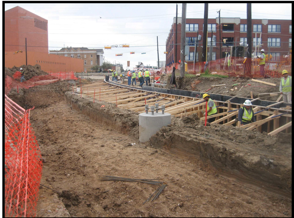
Forming & Excavating Header at Northbound Good Latimer
