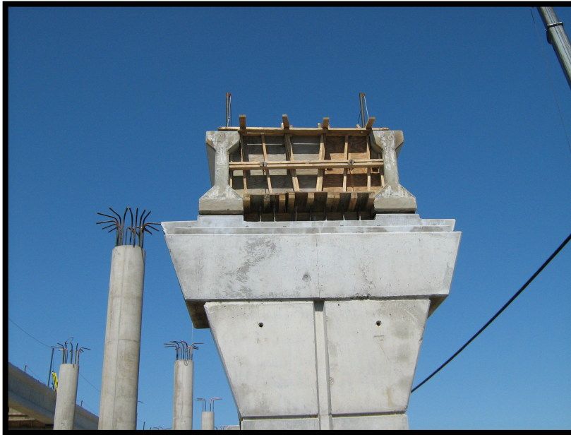
NW-3: Pier Diaphragm
