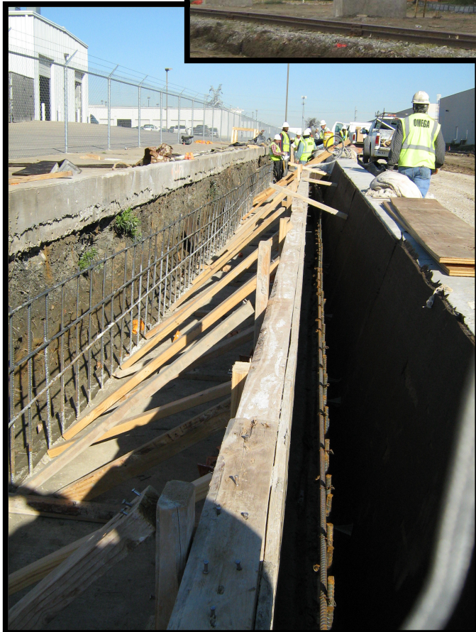
NW-4: Sub-ballast Wall North of Trinity Mills Road
