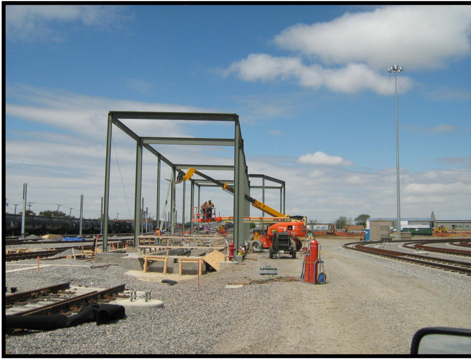
Steel Erection for SLRV Wash Building
