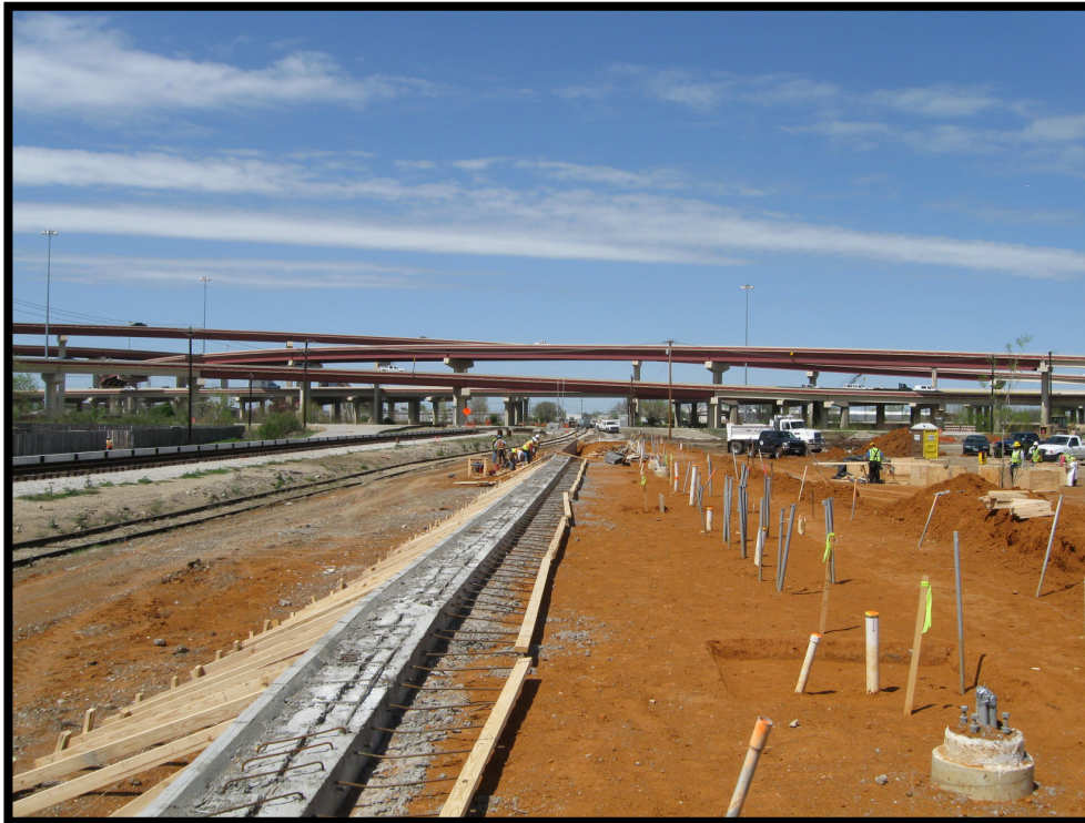
NW-4: Trinity Mills Station Northbound Platform Grade Beam
