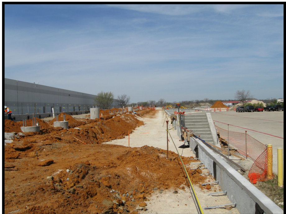
NW-4: North Carrollton/Frankford Station Select Fill Installation
