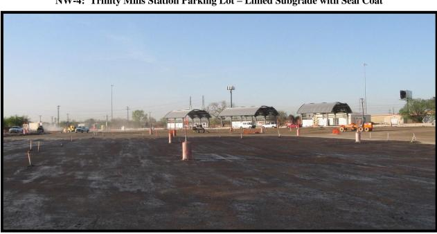
NW-4: Trinity Mills Station Parking Lot – Limed Subgrade with Seal Coat
