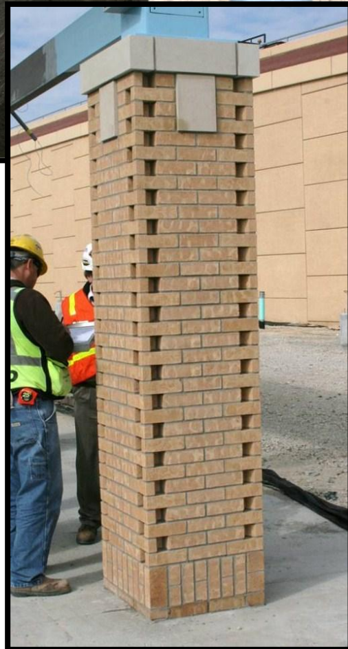
University of Dallas Station – Column Cladding
