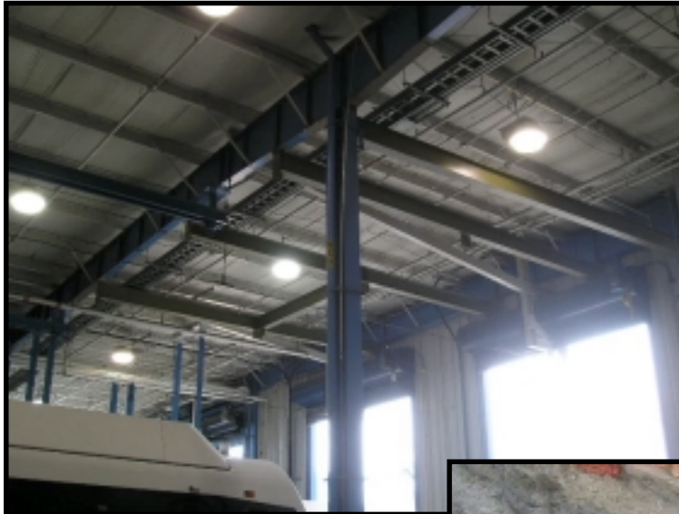
New Structural Steel Framing at Running Maintenance Bay
