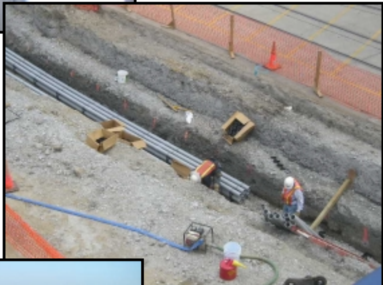
Ductbank Installation
