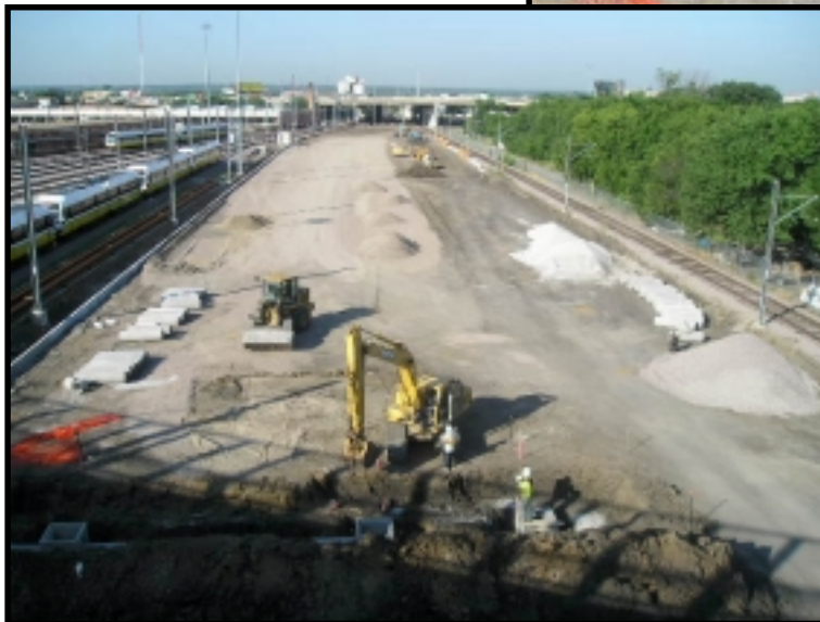
Sub-ballast Installation at Storage Track Yard Area
