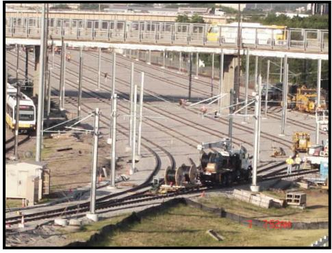
Signal Wire Truck Moving into New Storage Track Area
