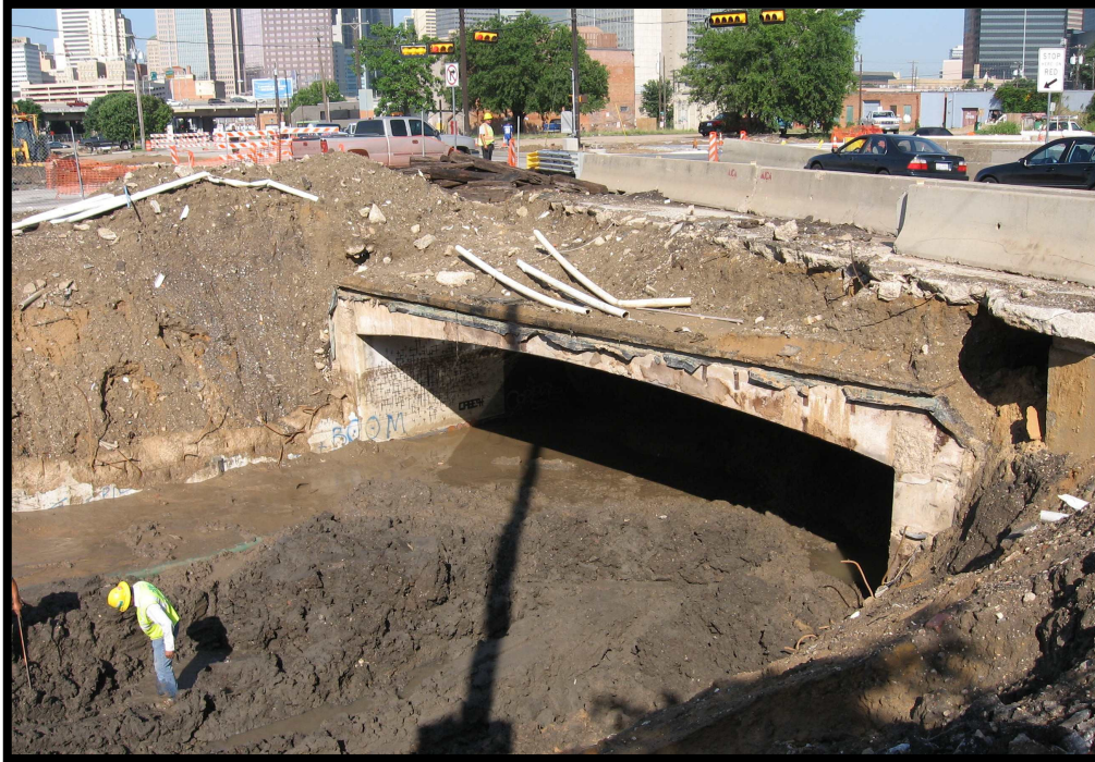
SE-1: Good Latimer Tunnel Backfill
