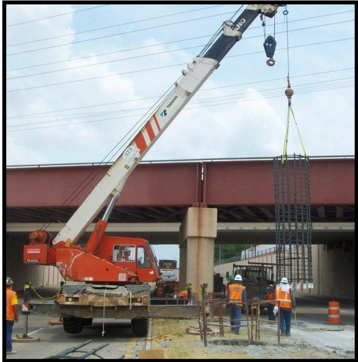
SH 78 Drilled Shaft Installation
