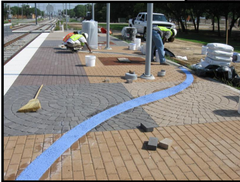
NW-3: Placement of Terrazzo at Farmers Branch Station
