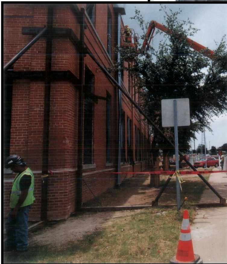
Supports for Building Exterior
