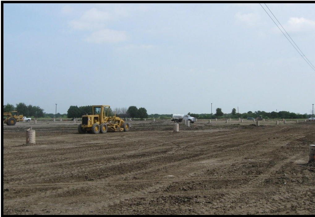
Grading & Light Pole Foundations
