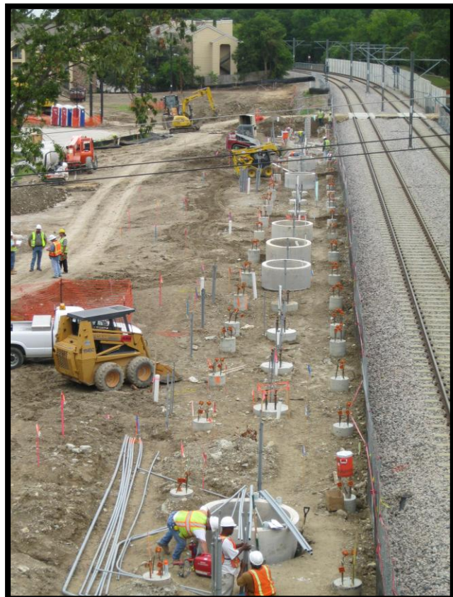
Station Platform Piers on West Side
