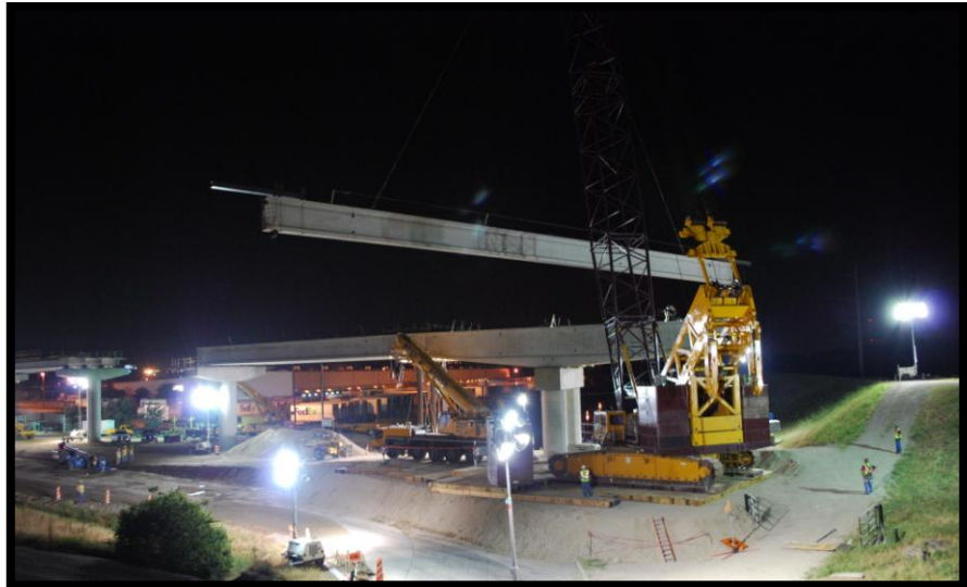
160' Precast Beams over Trinity River Levee
