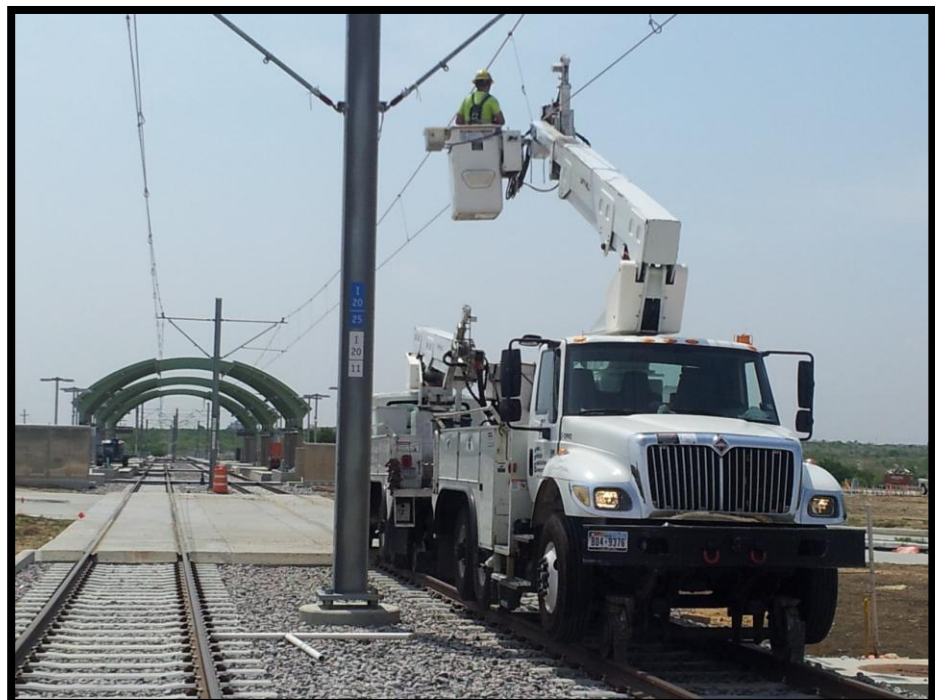
OCS Installation near Belt Line Station
