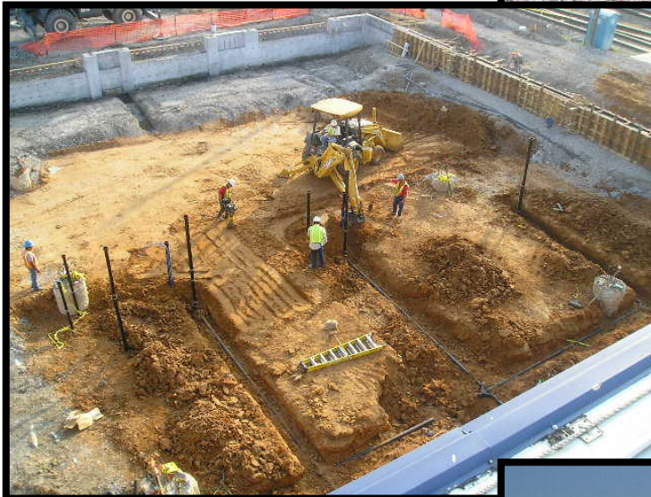
Grade Beam Formwork and Plumbing Rough-In for the Running Maintenance Addition
