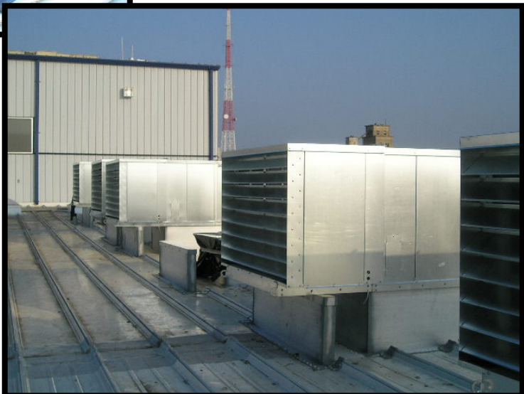
Air Handlers Installed on the Existing Running Maintenance Shop
