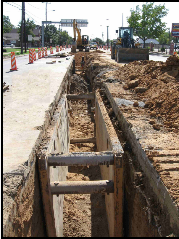
Water Main Installation in MLK Blvd.
