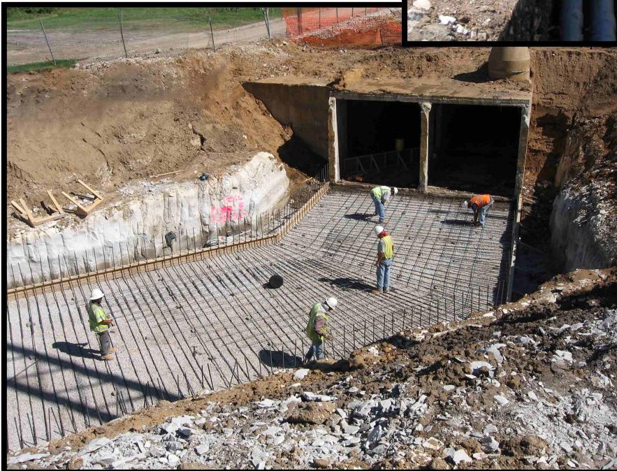
Steel Placement for Footing of Box Culvert at Peak's Branch
