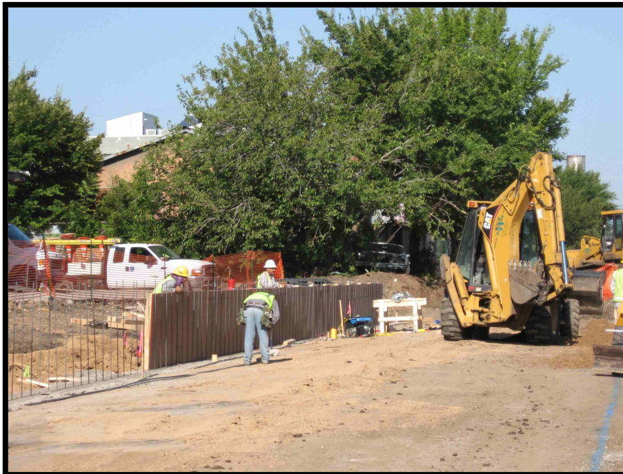
Ballast Wall Installation
