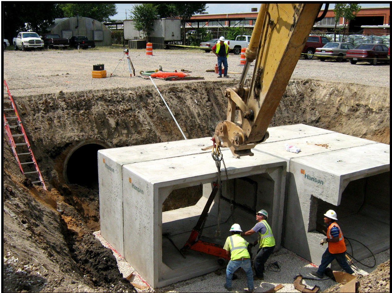
NW-2: Box Culvert Installation
