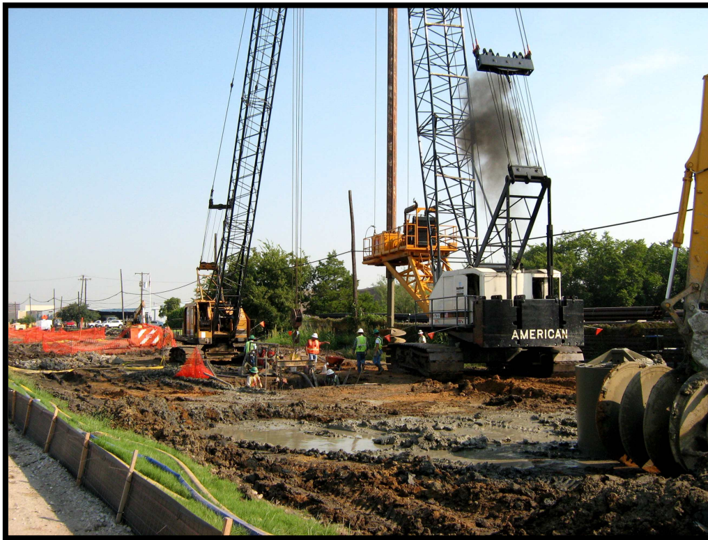
NW-3: Drilled Shaft Installation
