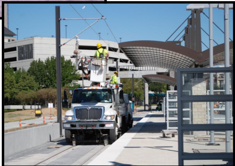
Stringing Overhead Catenary Cable at Las Colinas Urban Center Station
