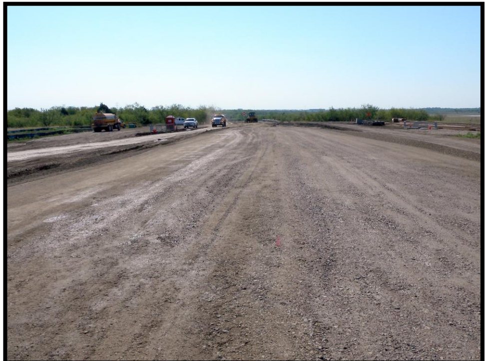
I-3 Alignment with Subballast
